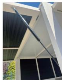
Gate switch, hydraulic rod for smoke test
